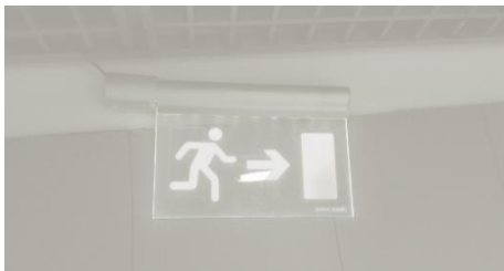
Back-up fire protection
